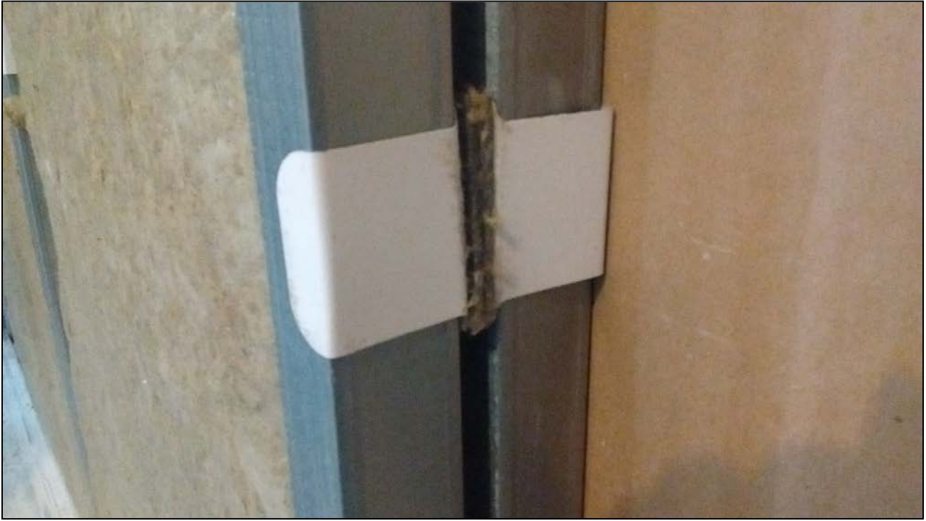
Sound Termination Clip attached to 1 5/8" Stud
